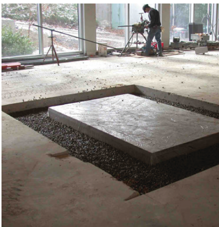
Figure 1. Separated Slab: The slab has been designed and implemented at customer site based on initial comprehensive site survey data.
