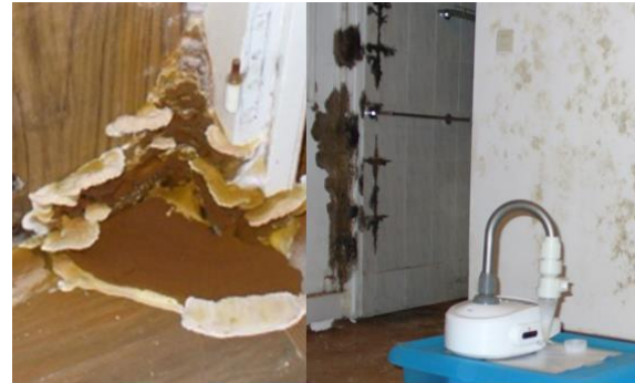
Figure 1: Extensive spreading of Serpula lacrymans mycelium.
