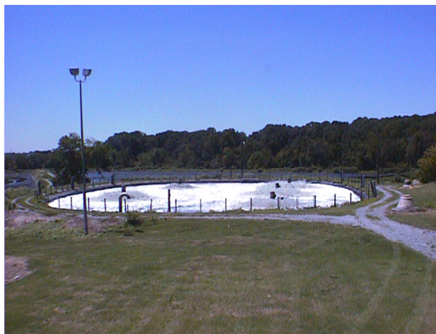
Pre-treatment pool: Before effluent is discharged from the facility it must be treated in one of these pools.
