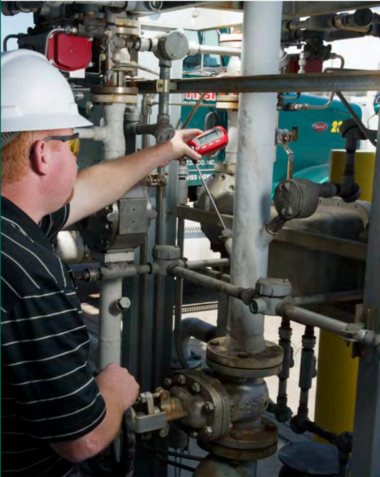
It's not always possible or practical to remove instruments from a process for calibration. In situ verification at a single point may be the only way to know whether an instrument is performing as expected. A single point verification is most effective over a narrow temperature range and when combined with other trends and information related to the process and equipment. It also requires the process not to be in a dynamic state of change.
