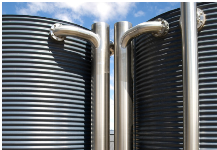
Tanks in the sun: Various surface materials were used for water tanks to establish maximum thermal efficiency.
