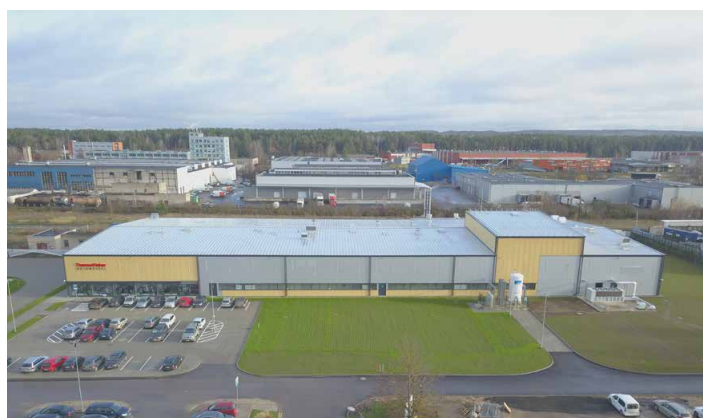
Figure 2. Construction of the manufacturing site in Vilnius, Lithuania.
