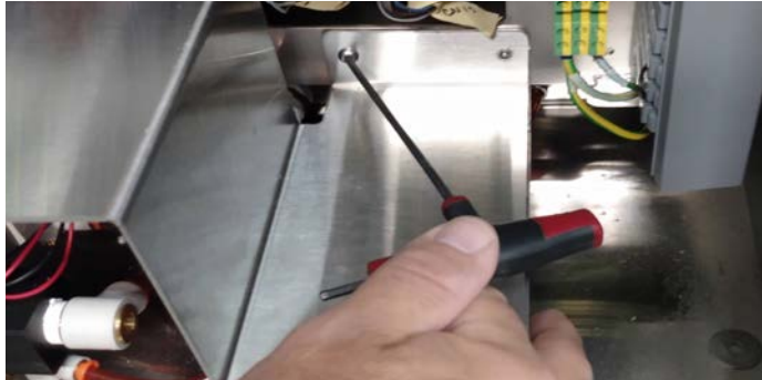
Figure 3.61. Removing the plate that covers the large valve.
