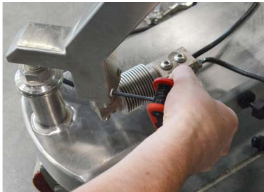
Figure 3.54. Replacing the bolts securing the load cell to a leg.
