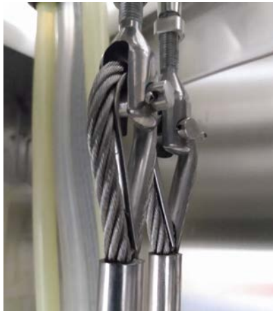
Figure 3.72. Top end of the 1/4 in. cables.
