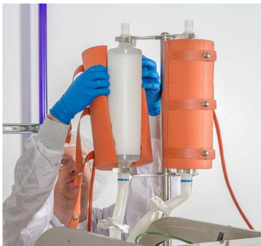
Figure 3.67. Installing heaters.
