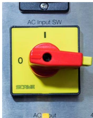
Figure 3.5. Main power switch shown in “off” position.
