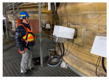
Use of continuous monitoring system for mercury emissions in a coal-fired thermal power plant
