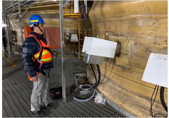
Use of continuous monitoring system for mercury emissions in a coal-fired thermal power plant
