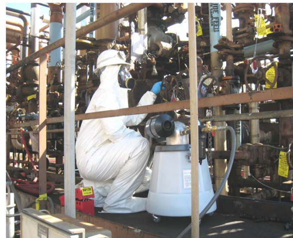
Mercury clean up. PSC worker using “special” mercury vacuum on flange.
