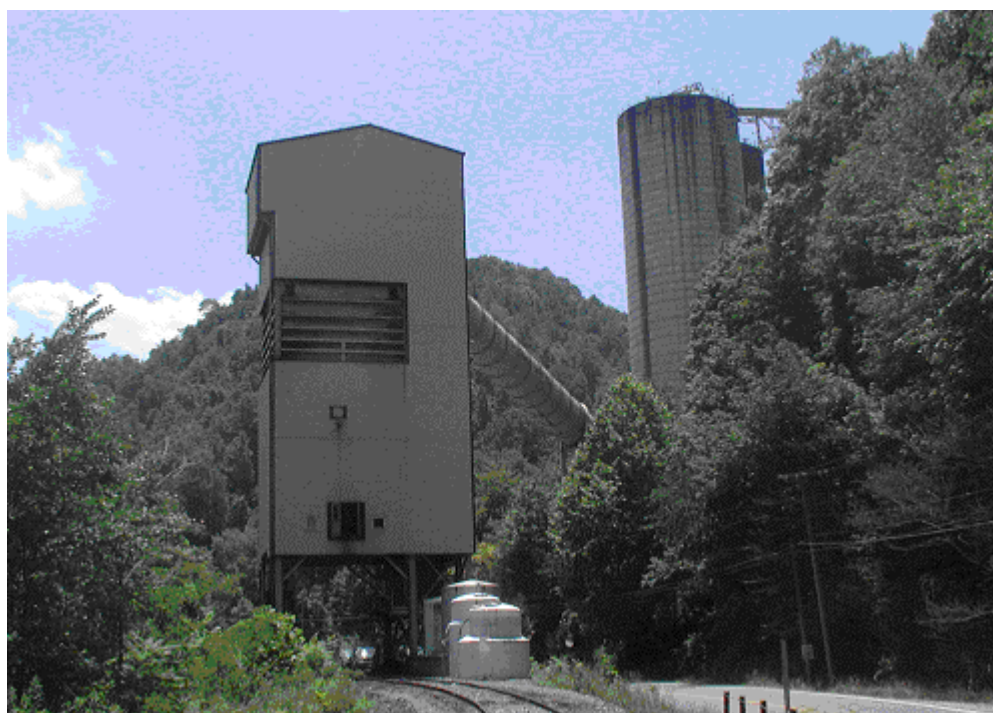
Figure 3. Loadout silos and loadout tower at Toms Fork.
