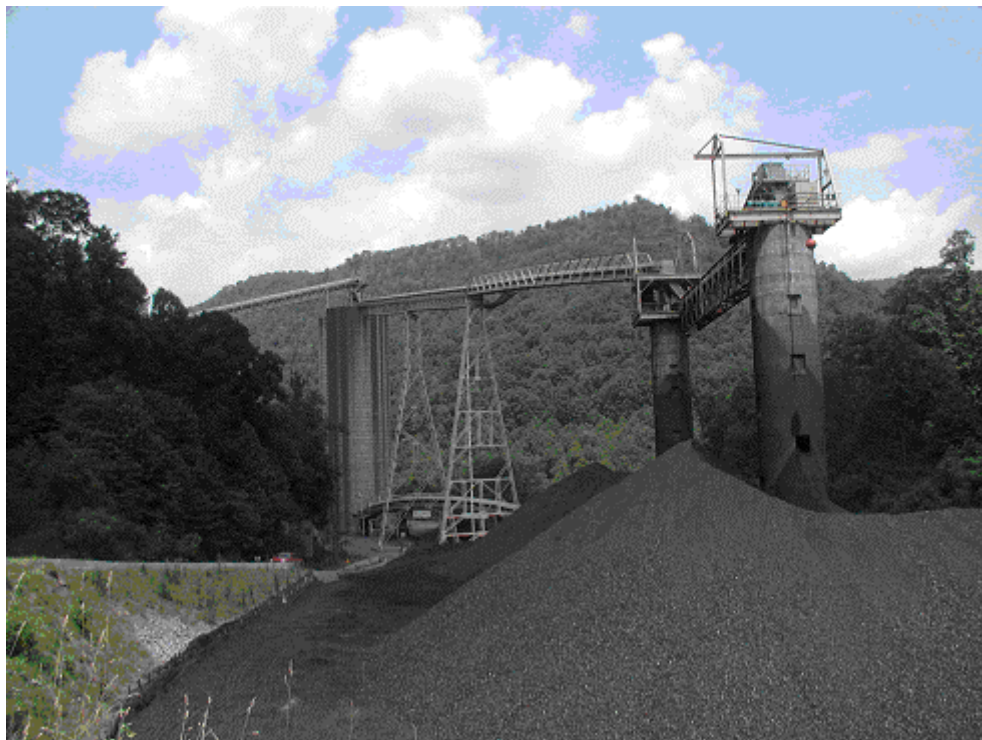
Figure 2. Stacking tube stockpiles at Toms Fork Loadout
