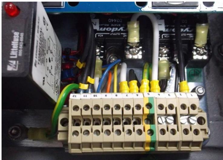
**Figure 3–6.** Purge Control Unit TB1 & Grounding Lug
