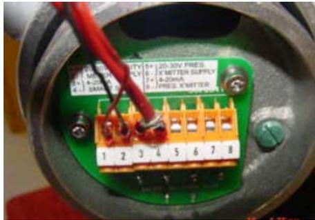
**Figure B-2.** Sarasota FD910 headmount assembly terminal connections
