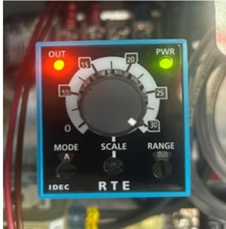
**Figure 10–3.** Timer relay in normal operation with default setting of 30 minutes
