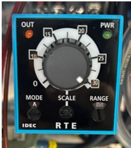
**Figure 10–4.** Timer relay during loss of purge pressure prior to supply restoration
