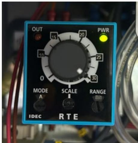
**Figure 10–5.** Timer relay during 30 minute timer countdown
