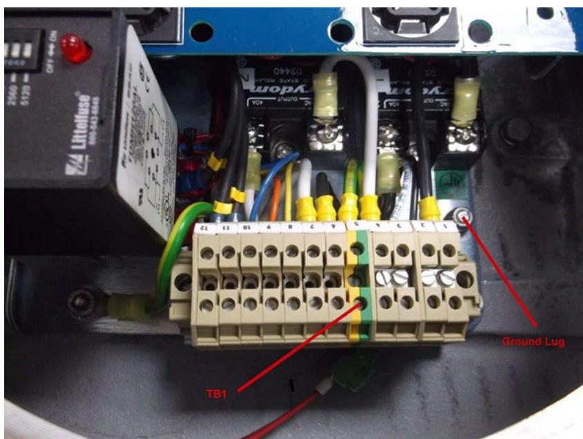
**Figure 10–2.** Purge Control Unit TB1 and Grounding Lug
