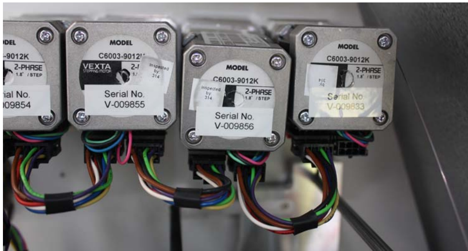
Figure 159. Cables connected to valves
