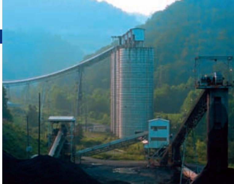
Coal storage tower
