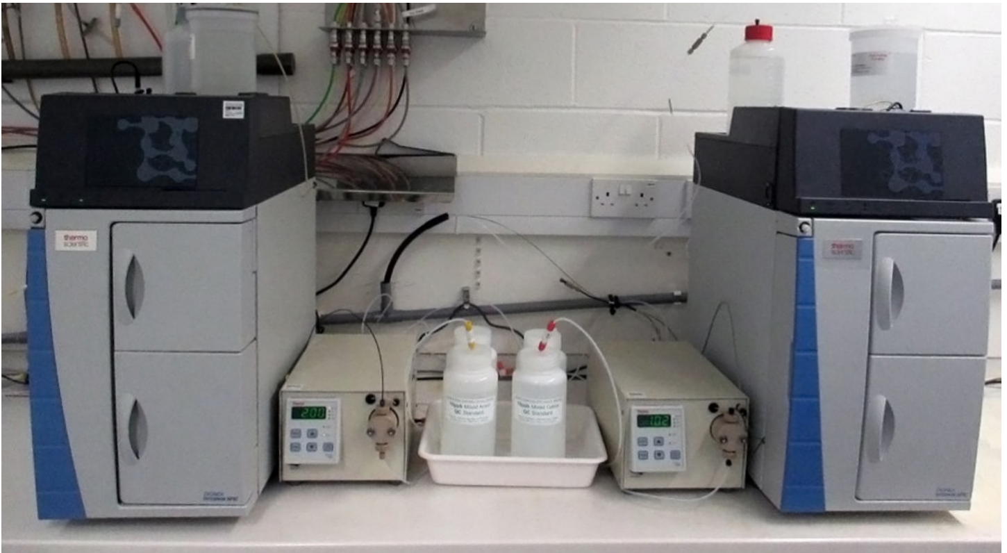
Figure 4. At the Sizewell B Nuclear Power Plant Chemistry Lab, Dionex Integrion HPIC systems are dedicated to the analysis of either cations or anions in condensate samples. Photo courtesy of EDF.
