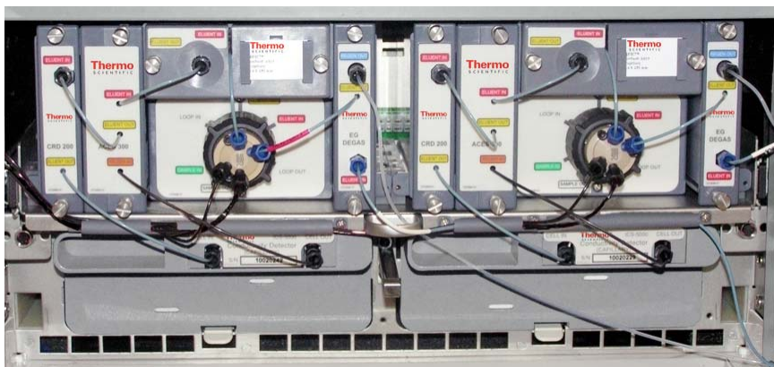
Figure 3-68. Completed Dionex IC Cube Plumbing for a Dual Conductivity Detection System
