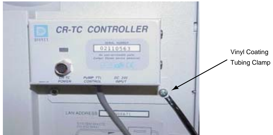
Figure 7 Placement of Upper Vinyl Coated Tubing Clamp
