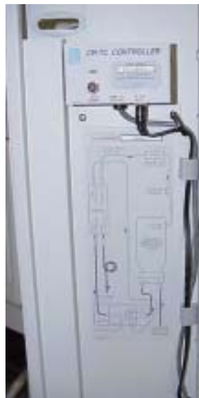
Figure 10 The Power Supply DC 24 V Cable and Pump TTL Control Cable Routed through the Chase and Upward Along the Door to the Controller
