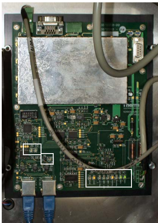
Figure 1-33. Temperature Controller board
