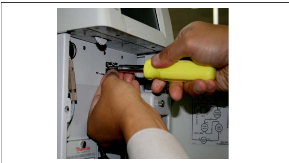
Figure 2. Installing the ER1 Column Bracket Clip
