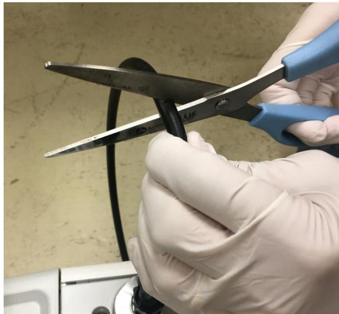
*Figure 28: Trimming the hose*
