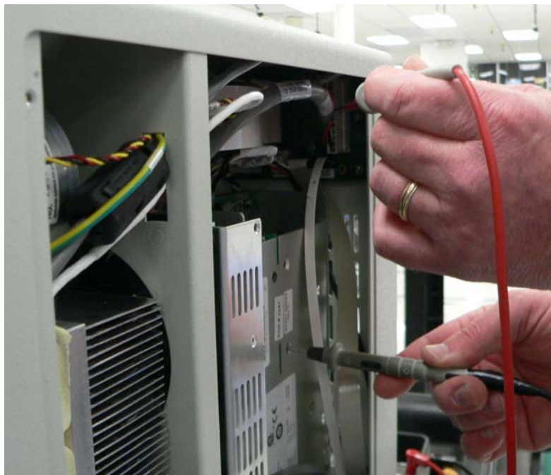
Figure 205. Checking the DC voltage output of the logic voltage power supply
