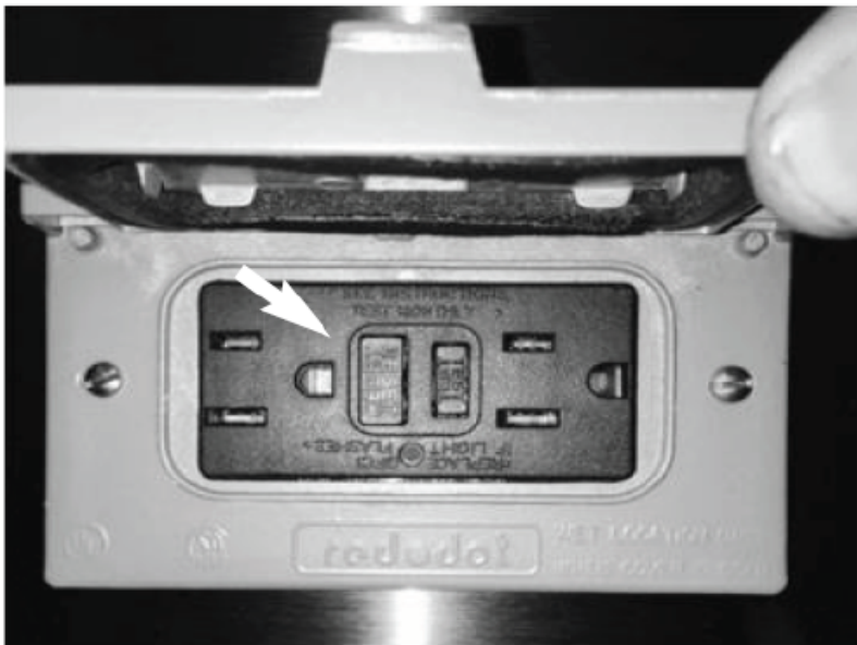
Figure 31. Reset Button on GFCI Outlet
