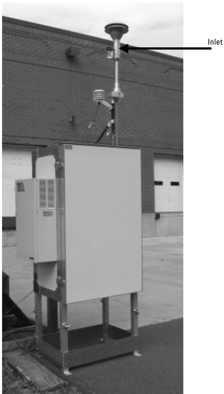
Figure 2-31. Outdoor enclosure with inlet installed.
