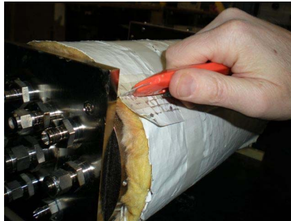
Figure 5–42. Cutting Insulation Paper at the Seam
