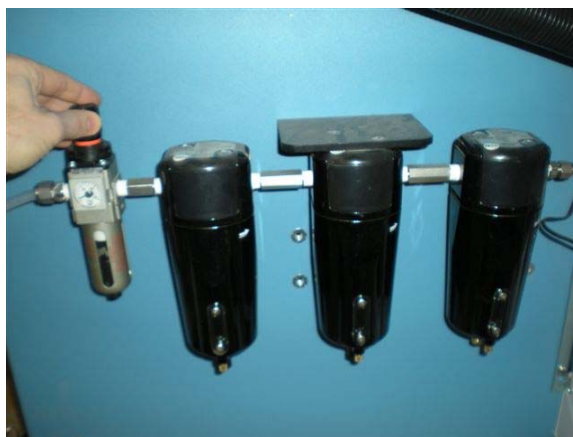
Figure 5–18. Turning Off House Air
