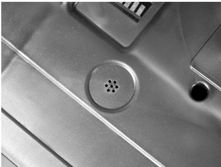
Figure 5–40. Battery compartment vent
