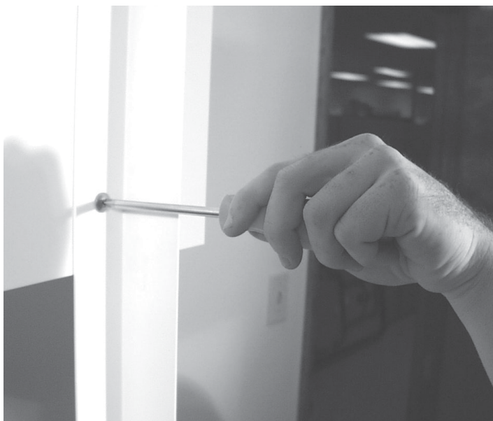
Figure 2-45. Be sure to hold the screw with a screwdriver while turning the nut.
