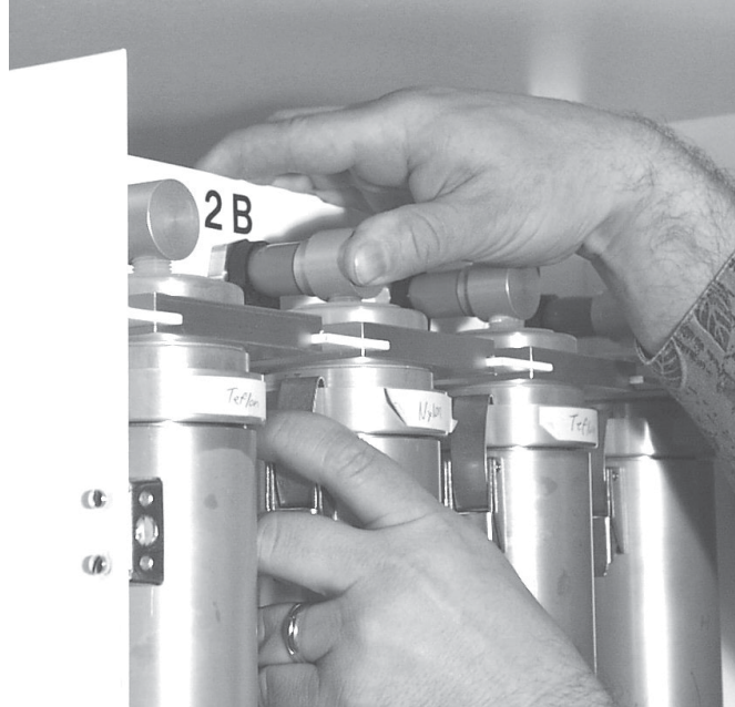
Figure 4-22. Manually securing the hose connection.
