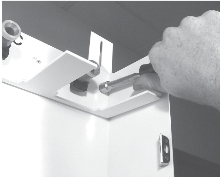
Figure 2-17. Securing the top of the shelter box to the leg studs.
