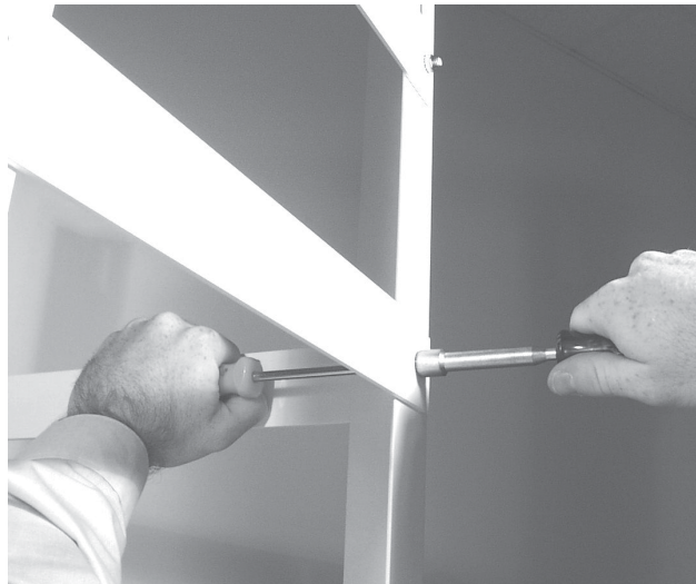
Figure 2-15. Securing a bottom side bracket plate to the shelter legs.
