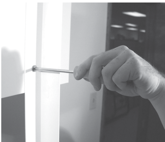
Figure 2-20. Holding the screw with a screwdriver while turning the nut.
