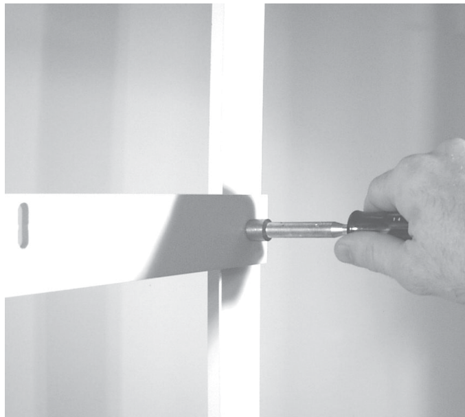
Figure 2-11. Securing the hose assembly mounting plate to the shelter legs.
