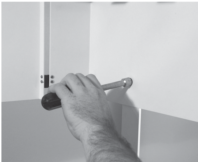
Figure 2-19. Securing the bottom of the shelter box.
