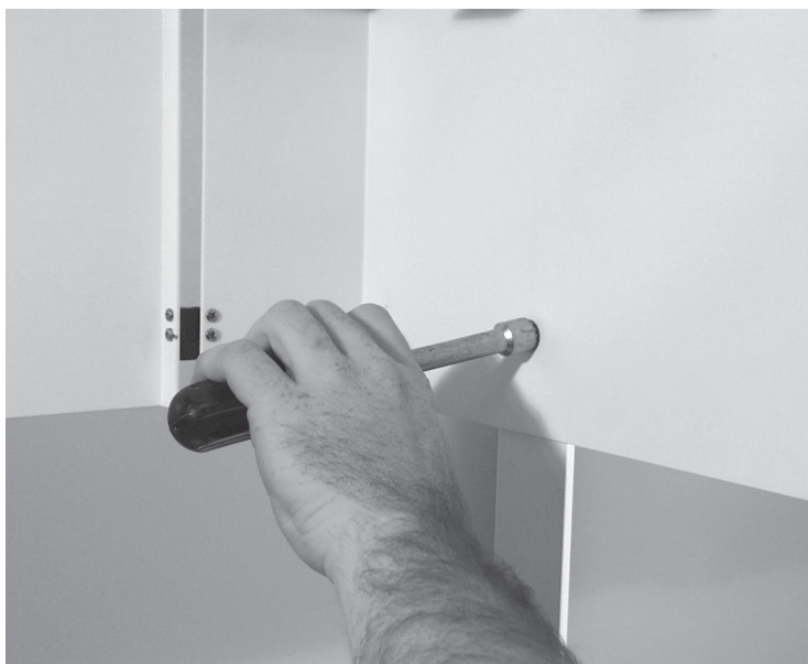
Figure 2-44. Securing the bottom of the shelter box.
