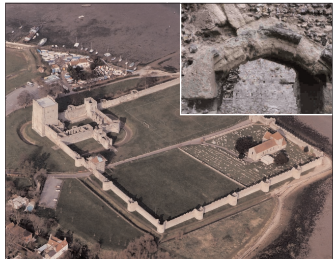
Figure 1. Portchester Castle: a historic monument suffering stone biodeterioration. Figure 2 (inset). Stone decay and crusts on decorative arches at Portchester Castle.
