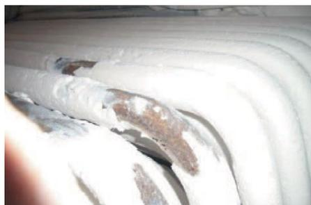
Figure 2. Boiler tubes coated with SiO<sub>2</sub>.
