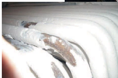
◀ Figure 2 Boiler tubes coated with SiO 2 .
