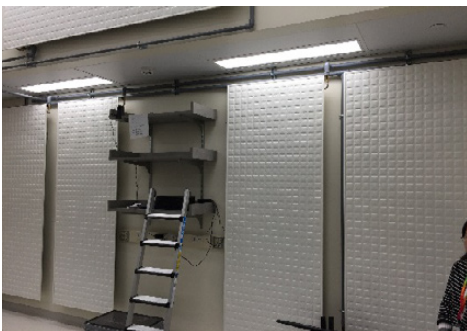
Chilled water panels
